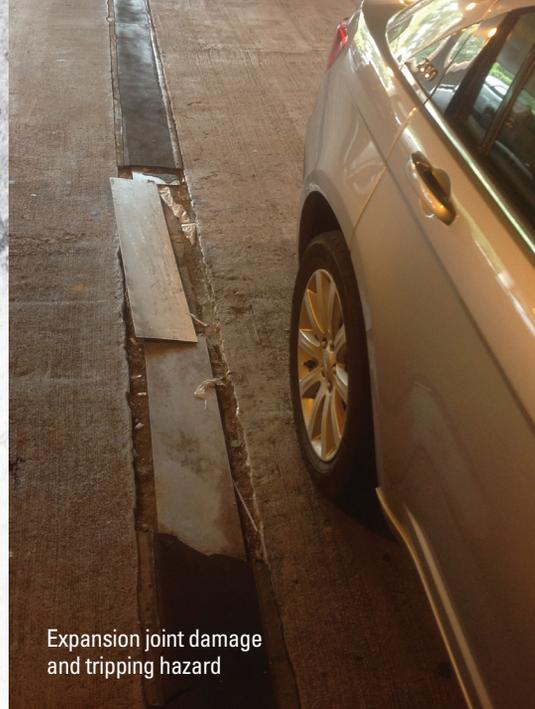
Expansion joint damage and tripping hazard
