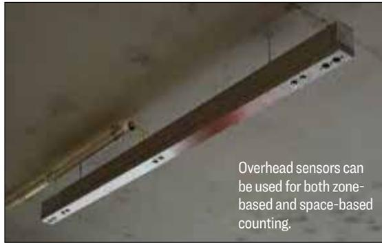
Overhead sensors can be used for both zone-based and space-based counting.
